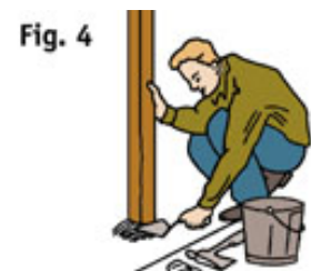
Build a mound around each post to eliminate standing water.
